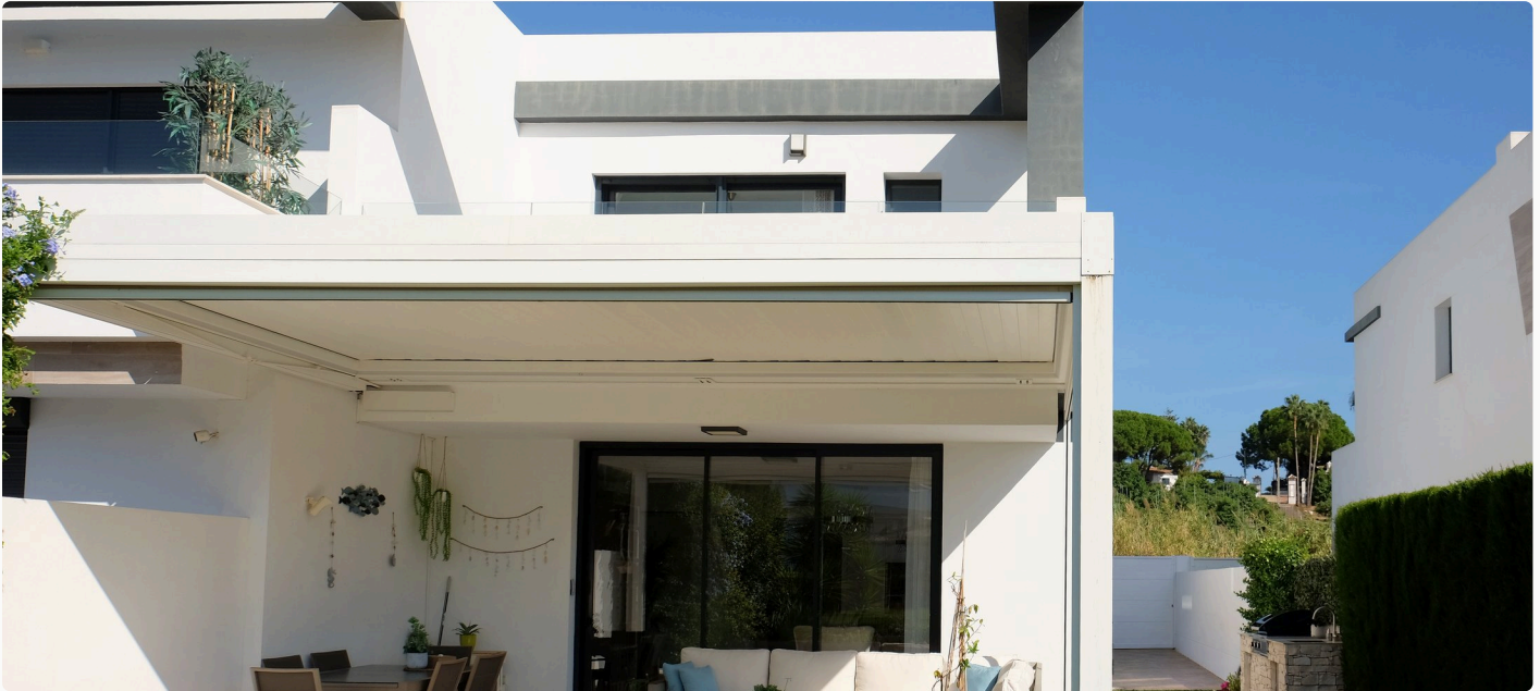
Covered terrace under the bioclimatic pergola
